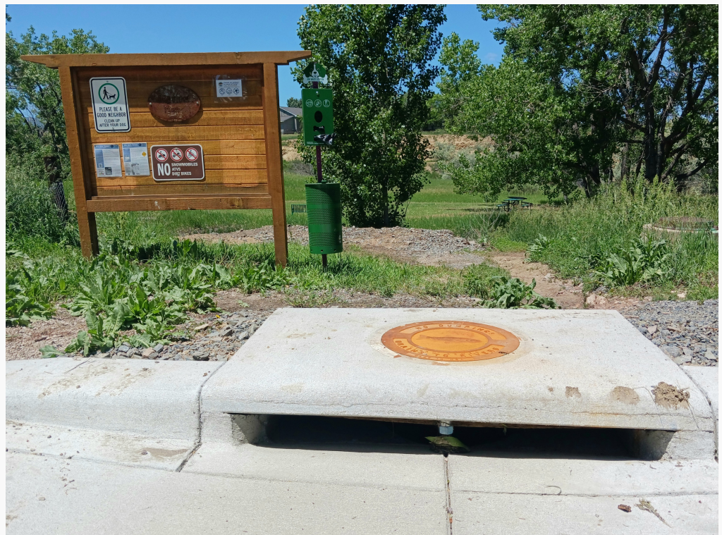
The new inlet, concrete work, and doggie clean-up station at the park entrance. Photo by Cindy Leikam
